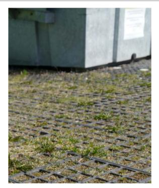
For more than 30 years, PURUS PLASTICS has manufactured ECORASTER® permeable ground reinforcement system, made of 100% recycled materials (LDPE). Our very first installation of ECORASTER E50 "Classic" was installed over 30 years ago at a busy waste collection depot. This specific installation is found in a cold climate and the grid has been subjected to the constant freeze-thaw cycle as well as constant snow plowing.
